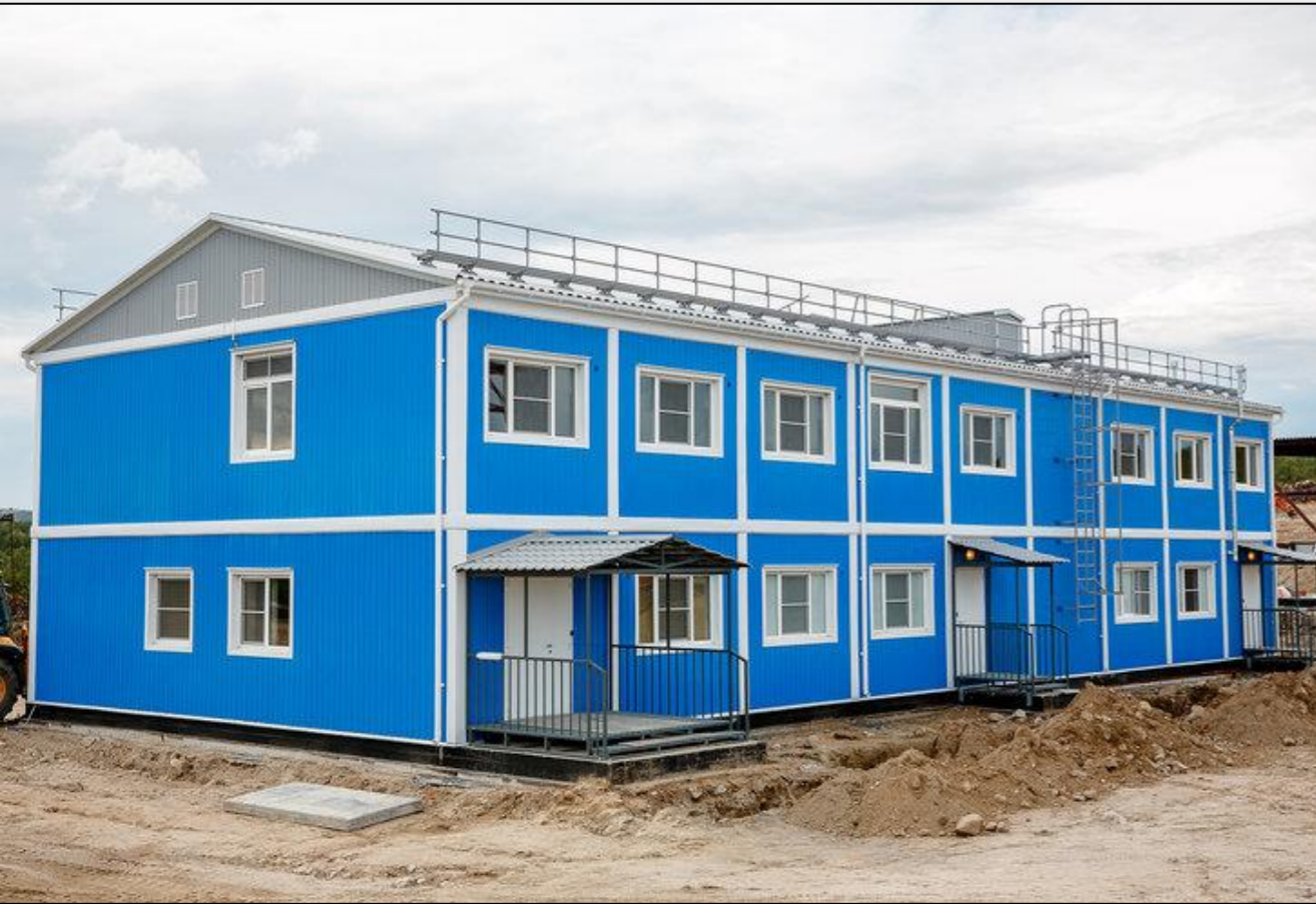
Administrative building of MSW recycling plant, Murmansk
